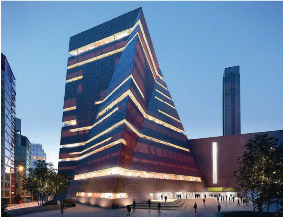
HERZOG & DE MEURON'S TATE MODERN EXTENSION WILL FEATURE A LATTICE BRICK FACADE THAT ALLOWS LIGHT TO SHINE THROUGH WHILE COMPLEMENTING THE SURFACE OF THE ORIGINAL GILES GILBERT SCOTT STRUCTURE. DUE TO BE COMPLETED IN 2016, THE NEW BUILDING WILL STAND AT 64.5M, ITS HEIGHT RESPONDING TO THE FORMER POWER STATION'S ICONIC 99M-HIGH CHIMNEY
